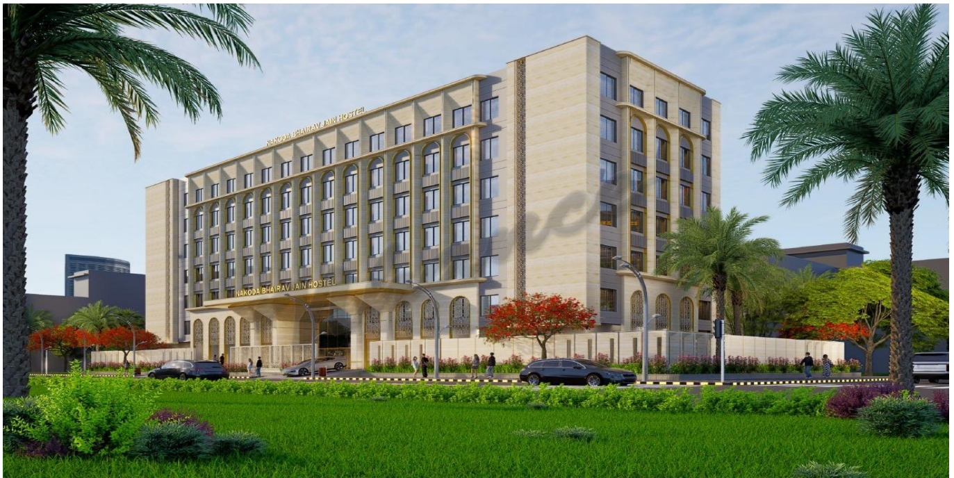
Nakoda Bhairav Boys Hostel, Jodhpur (Rajasthan)
