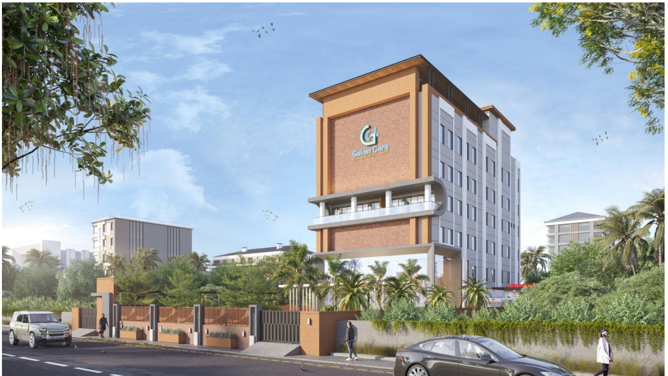
Galencare Hospital, Gandhinagar (Gujarat)
