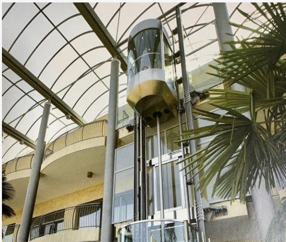
Supporting structure for lift
